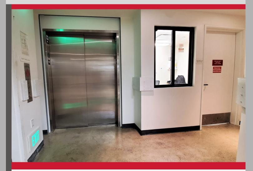
As shown above the same service elevator did not have enough swing clearance or a place to hold the smoke doors for this back of the house corridor floor. Instead the opening is being protected with an ICC-ES listed DSI 600 Elevator Smoke Containment System. Can you spot it?
