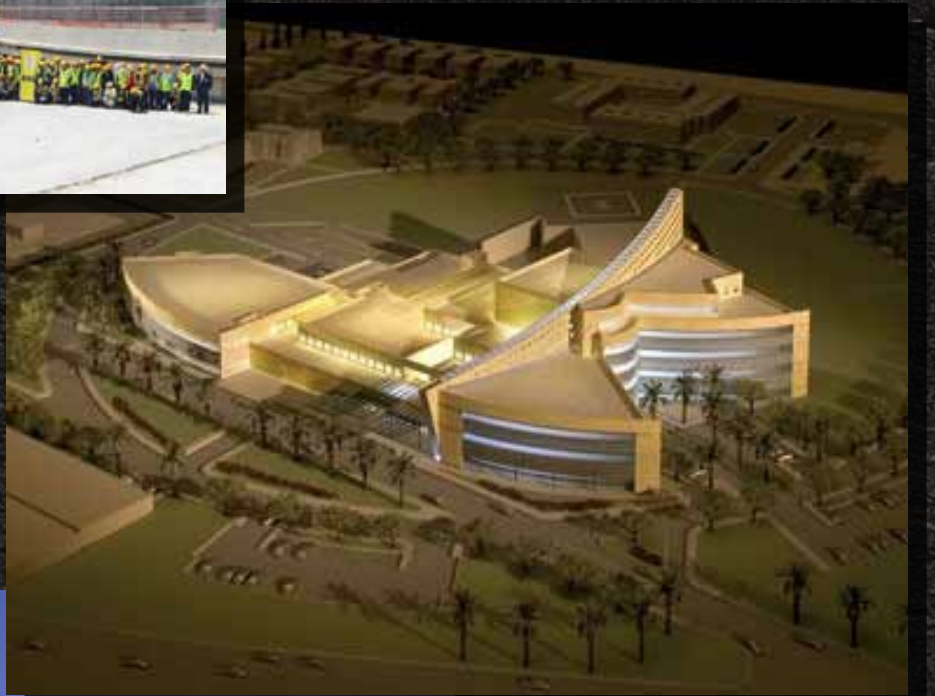
PRINCE HACHEM HOSPITAL, AQABA, JORDAN
